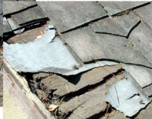
ASBESTOS CEMENT ROOF SHINGLES AND FELT (TAR PAPER)
